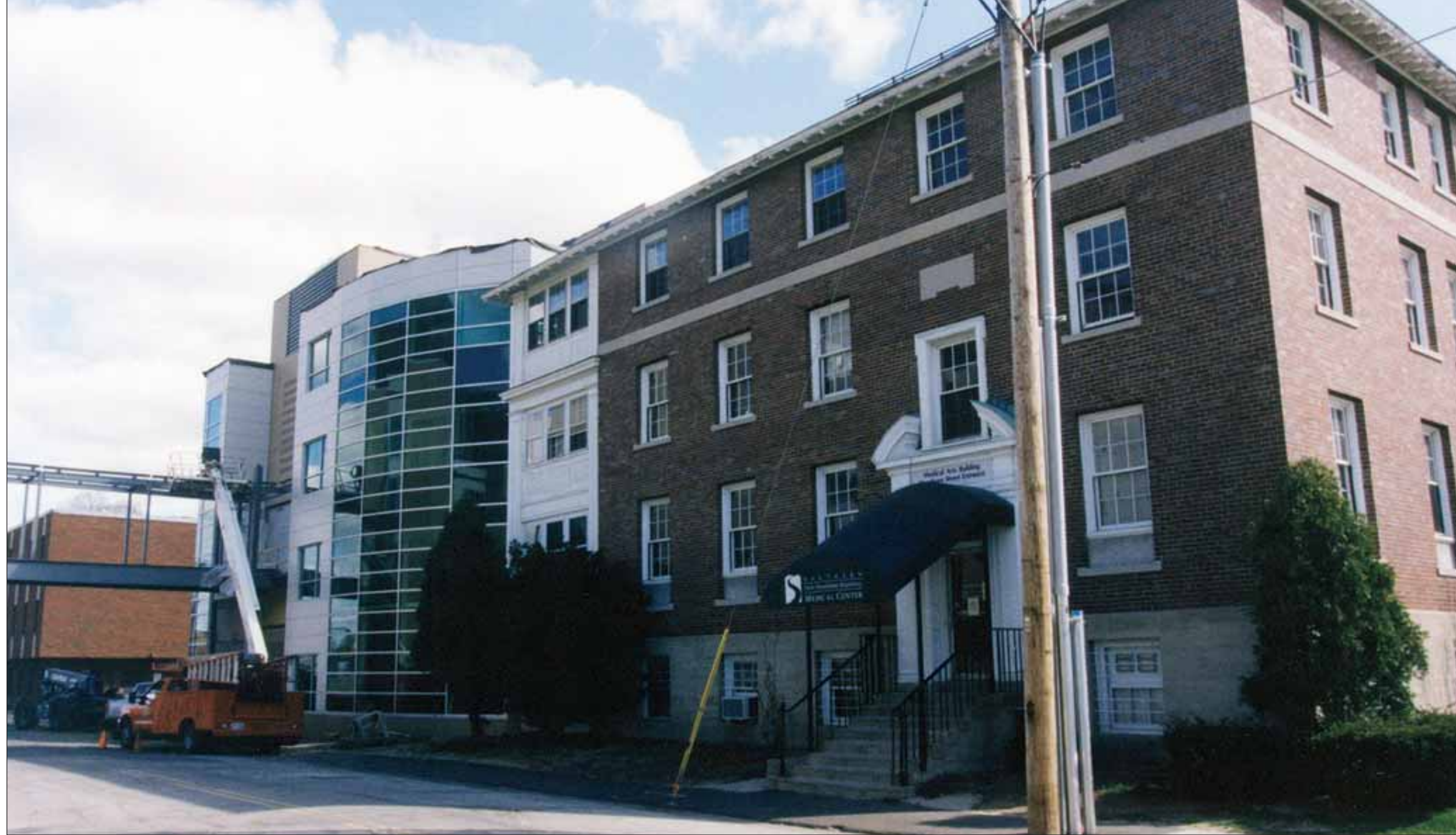
Construction of the new 10 Prospect Street Health and Education Building skywalk, 1999.
