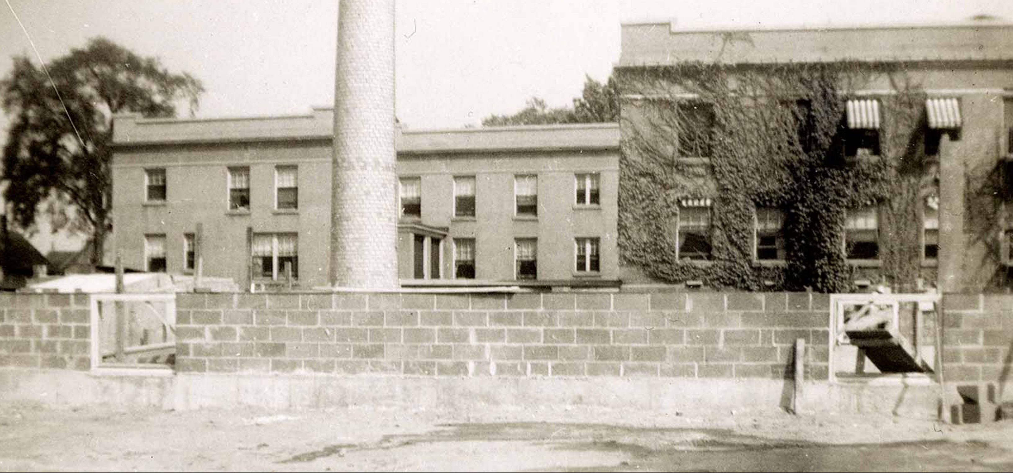
Construction continues on the new wing, 1958.
